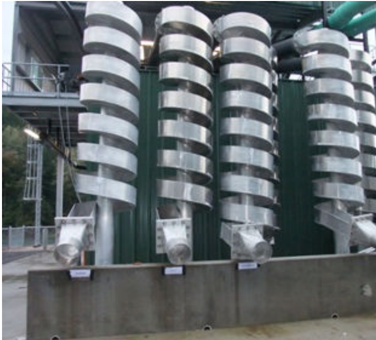
End of the line. Processed fish slide down spiral channels and into waiting baskets, totes etc. at the road level.
