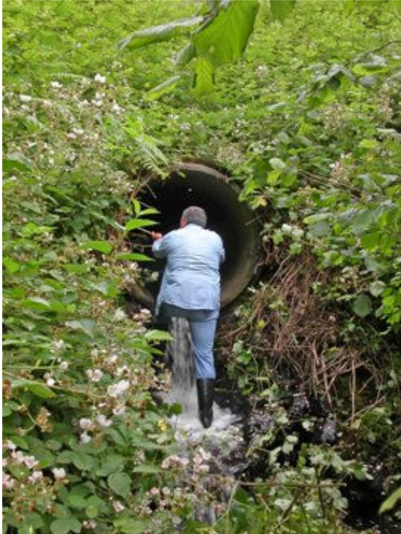
Photo: Willie Ck. Culvert, N. Fk. of Lewis
